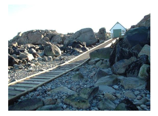
Owner: Town of York Project: Reconstruction of Nubble Lighthouse Boat Ramp Cost: \$108,810 Description: Reconstruction of a 140' timber boat ramp at a historic lighthouse. Ramp is founded on 8''x8'' posts installed on ledge with timber stringers epoxy anchored to ledge/large boulders. Work was completed during the winter of 2008/2009 and all
