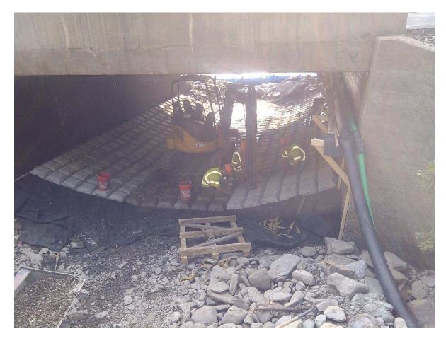
Owner: Maine DOT Project: Bridge Scour Countermeasures Cost: \$112,449 Description: Completed installation of concrete cable Mats in both Rumford, ME and Rangeley, ME. Projects included cofferdam installation, temporary stream bypass, excavation of existing streambed and installation of new concrete cable mat system, restoration of streambed. Status: Complete September 2013 Points of Contact: Gene Webb, MDOT (207) 577-8353
