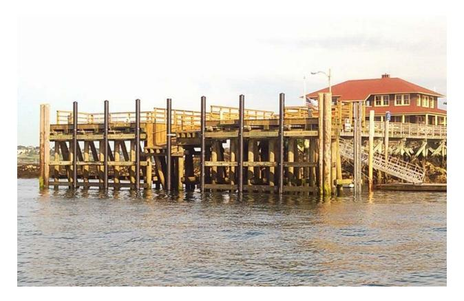
Owner: State of Maine Project: Casco Bay Timber Pier Rehabilitation Cost: \$1,068,000 Description: Expansion and Rehabilitation of 3 timber ferry docking piers, including installation of temporary berthing systems and replacement and upgrade of fendering systems. Status :Complete May 2013.
