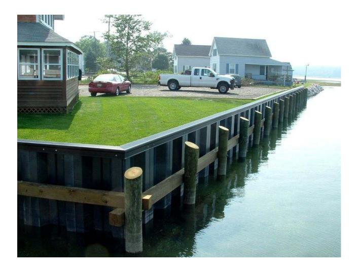
Owner: Bayley's Lobster Pound, Scarborough, ME Project: Bulkhead Replacement Cost: \$157,250 Description: Replacement of approximately 200' of failed timber bulkhead with new "Navy" style fiberglass sheetpile bulkhead. Project included demolition of the old bulkhead and installation of new helical anchor tiebacks. Status: Complete June 2008. Points of Contact: William Bayley (207) 883-4571
