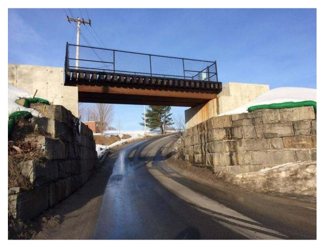
Owner: Maine DOT Project: Mallison Falls Road Railroad Bridge Rehabilitation Cost: \$335,495 Description: Replacement of an existing steel superstructure bridge with concrete abutments. Existing bridge and abutments were removed in their entirety. New abutments formed, poured and new bridge superstructure fabricated and installed. Project also included geofabric reinforced rail bed. Status: Complete December 2013 Points of Contact: Charlie Guy, MDOT (207) 557-9078
